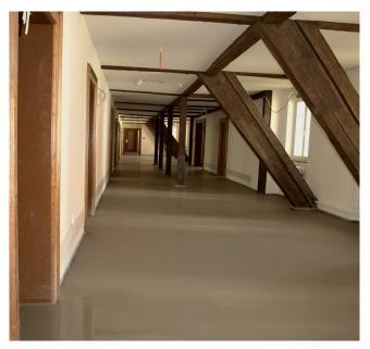
In this historical cloister area with a clinic operation UZIN NC 170 LevelStar was applied in different thicknesses on the most difficult substrates. The result is a perfect surface with optimal spread characteristics, and of course without any cracks.
